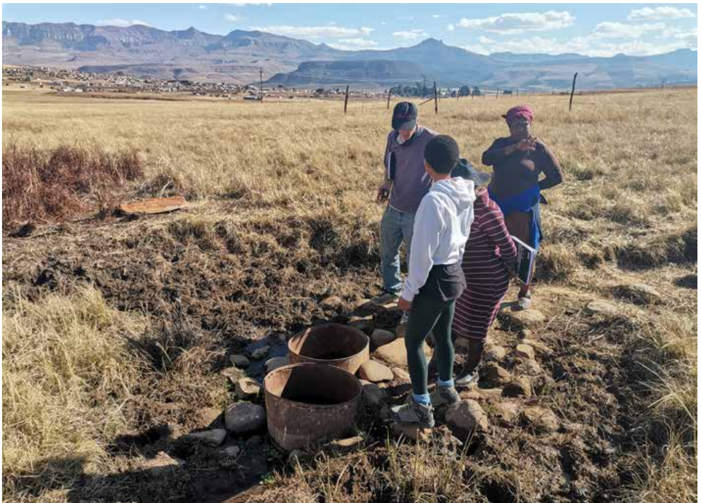
Initial visit to the spring to assess the existing infrastructure.
