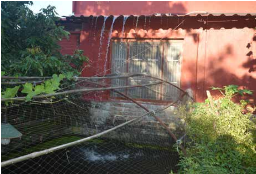
Rainwater harvested off a roof being captured in a fish pond.
