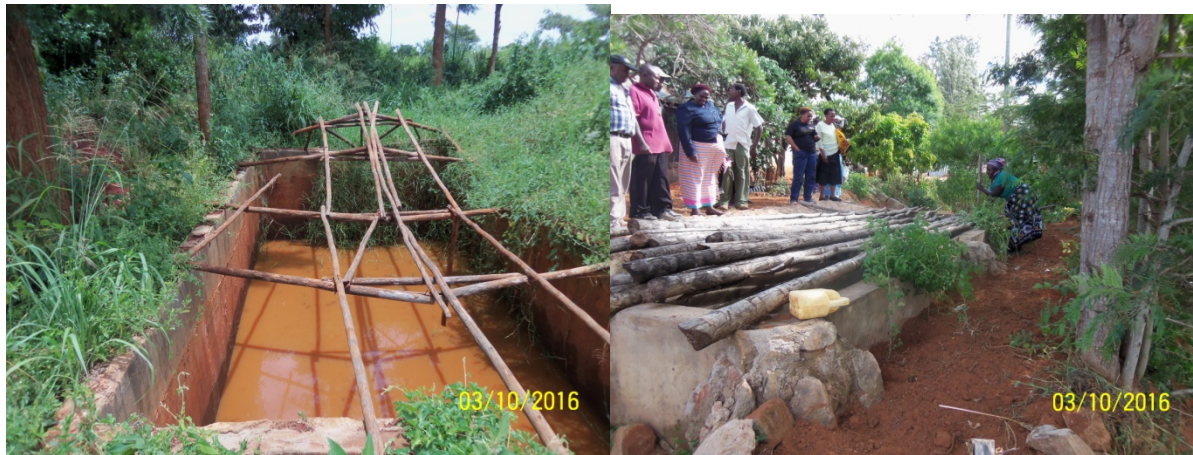
Figure 3: The picture of the right shows how a water-harvesting pit was adjusted by a woman farmer in Machakos who adopted it, covering it for safety and to reduce evaporation
