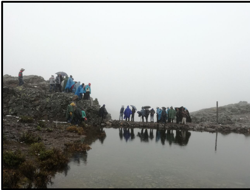
Figure 1: Farmers constructed three RWH systems of 8000 m 3 each
