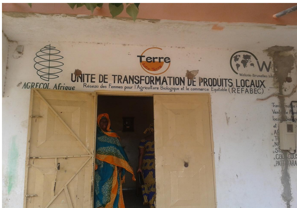
Photo 1: REFABEC agri-food processing unit
