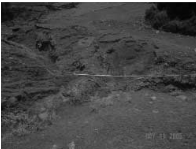
Taking the irrigation water across a 12.6 meter canyon using a eucalyptus log.
